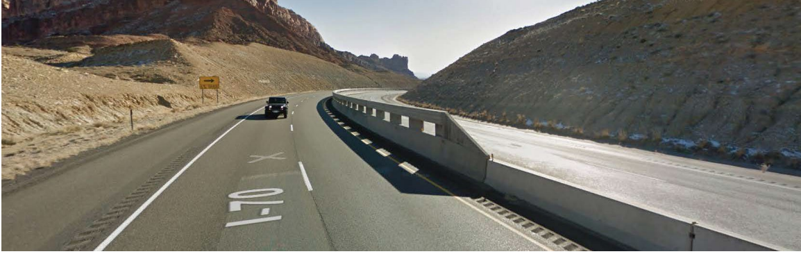
Figure 2.5 Utah DOT 84-in. Tall Roman Wall Installation [3]
